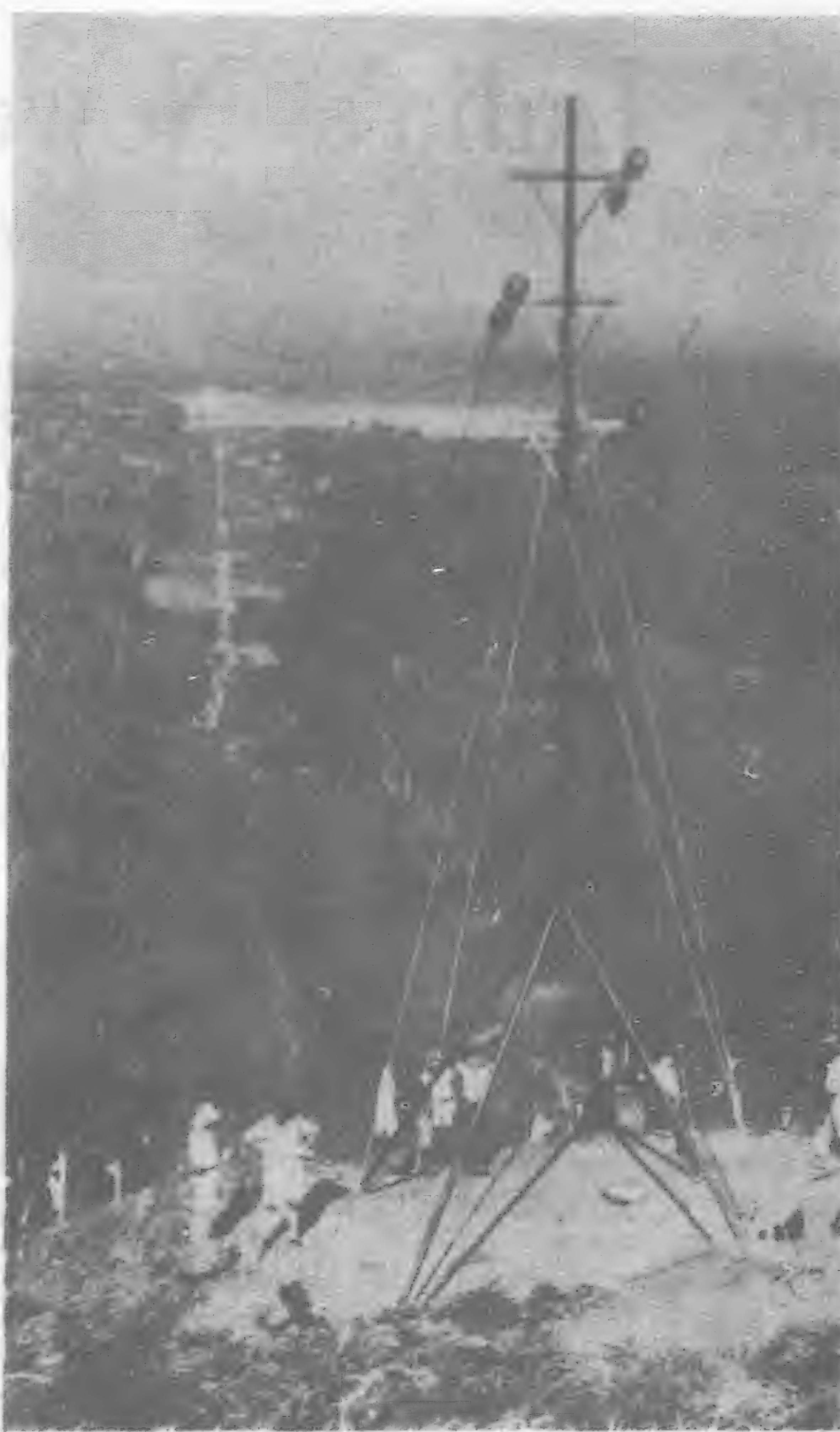
33,000 volts transmission line construction, Serdang loop line
